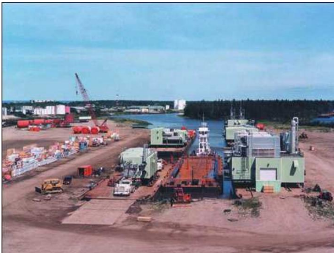
Figure 3. Oilfield Process and Accommodation Modules
